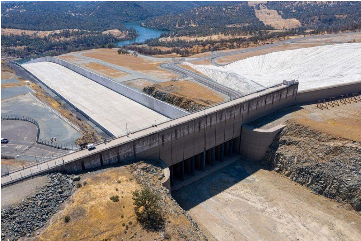
The Oroville Dam spillway at Lake Oroville during a drought in 2021. Photographer: David Paul Morris/Bloomberg
