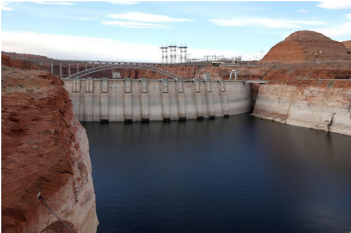
Lake Powell Falls To Lowest Level On Record Threatening Hydroelectric Power Production The Glen Canyon Dam at Lake Powell in Page, Arizona, on March 28. Photographer: Justin Sullivan/Getty Images
