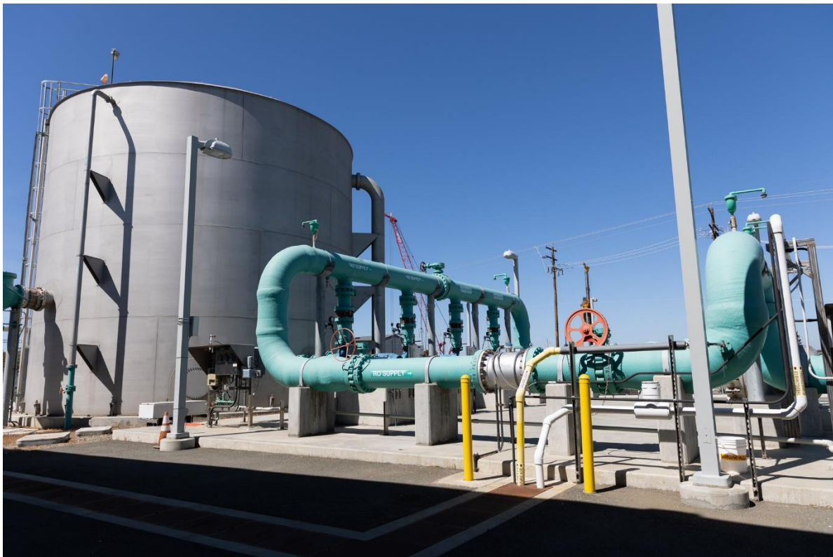
The 250,000-gallon inter-process tank that receives treated wastewater that has passed through the microfiltration treatment stage at the Silicon Valley Advanced Water Purification Center in San Jose on March 21, 2022. Photo by Magali Gauthier.
