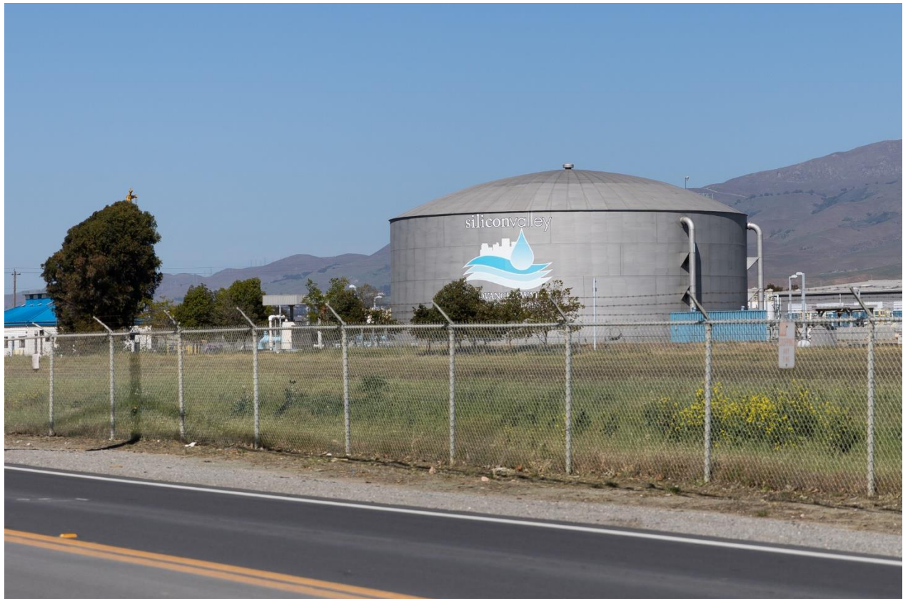
A 2.25-million-gallon metal holding tank at the Silicon Valley Advanced Water Purification Center in San Jose on March 21, 2022. Photo by Magali Gauthier.
